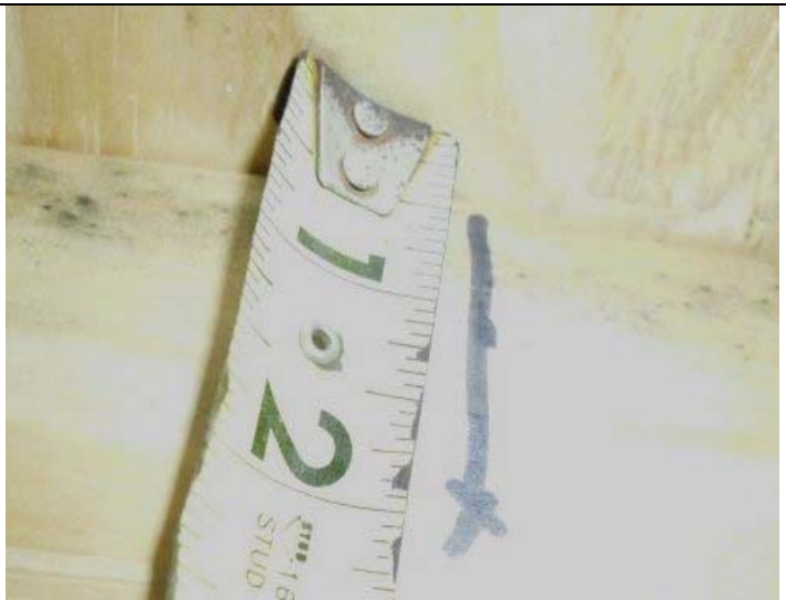
Roof deck attachment
