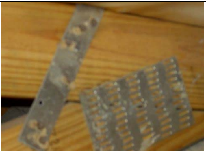
Roof to wall attachment
