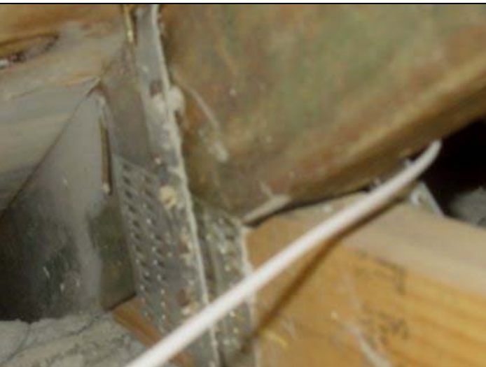
Roof to wall attachment
