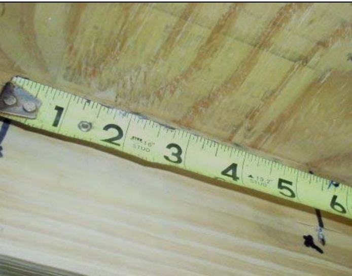
Roof deck attachment
